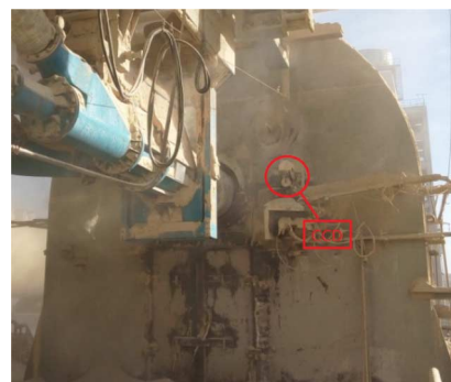
Fig. 2. CCD installation environment.
