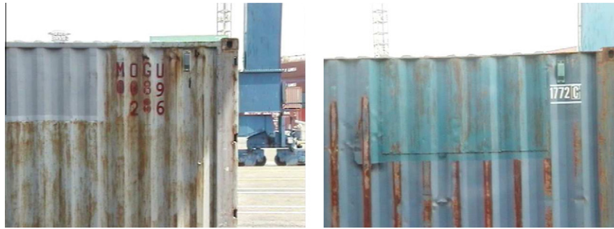
Fig. 22. Some failure examples of location.
